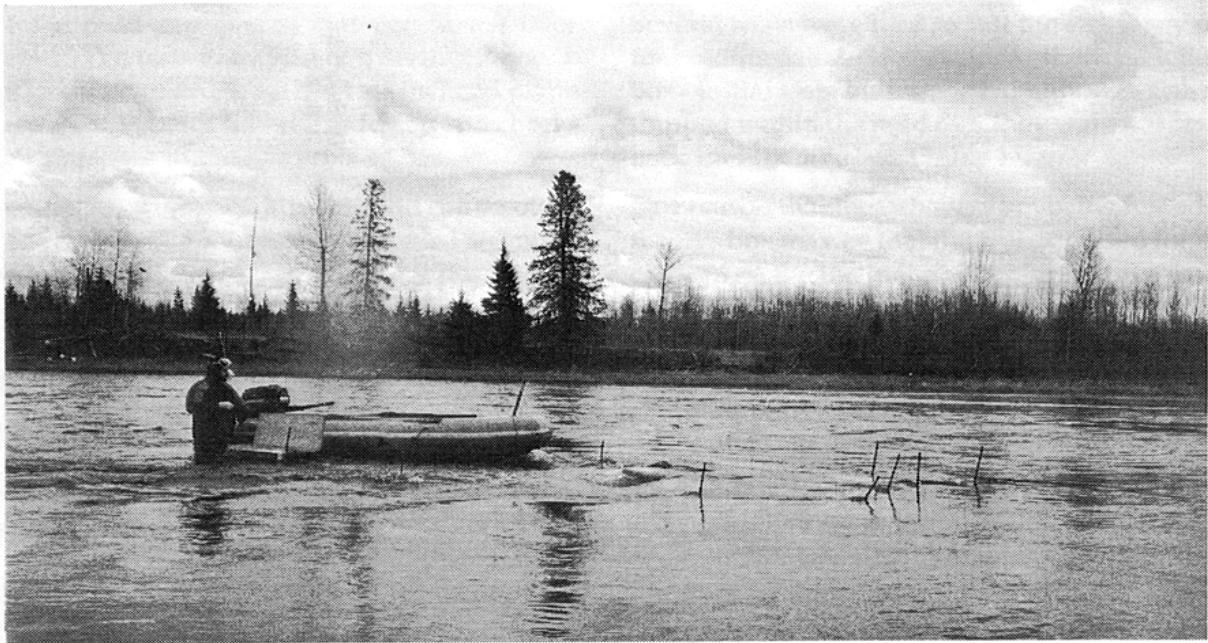
Plate 3: Floating Live Box Installation
