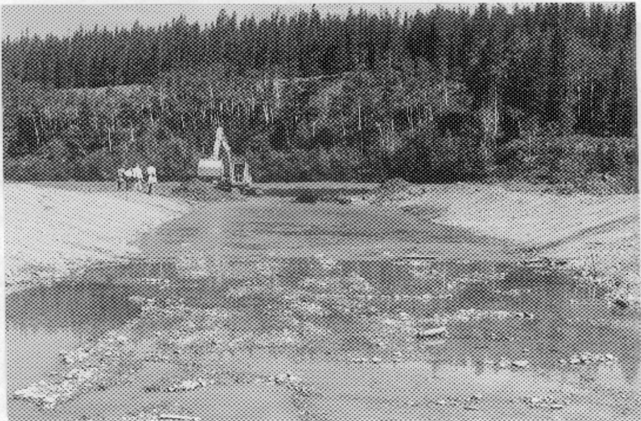
Photo 4: Excavation of Side Channel Using Backhoe
