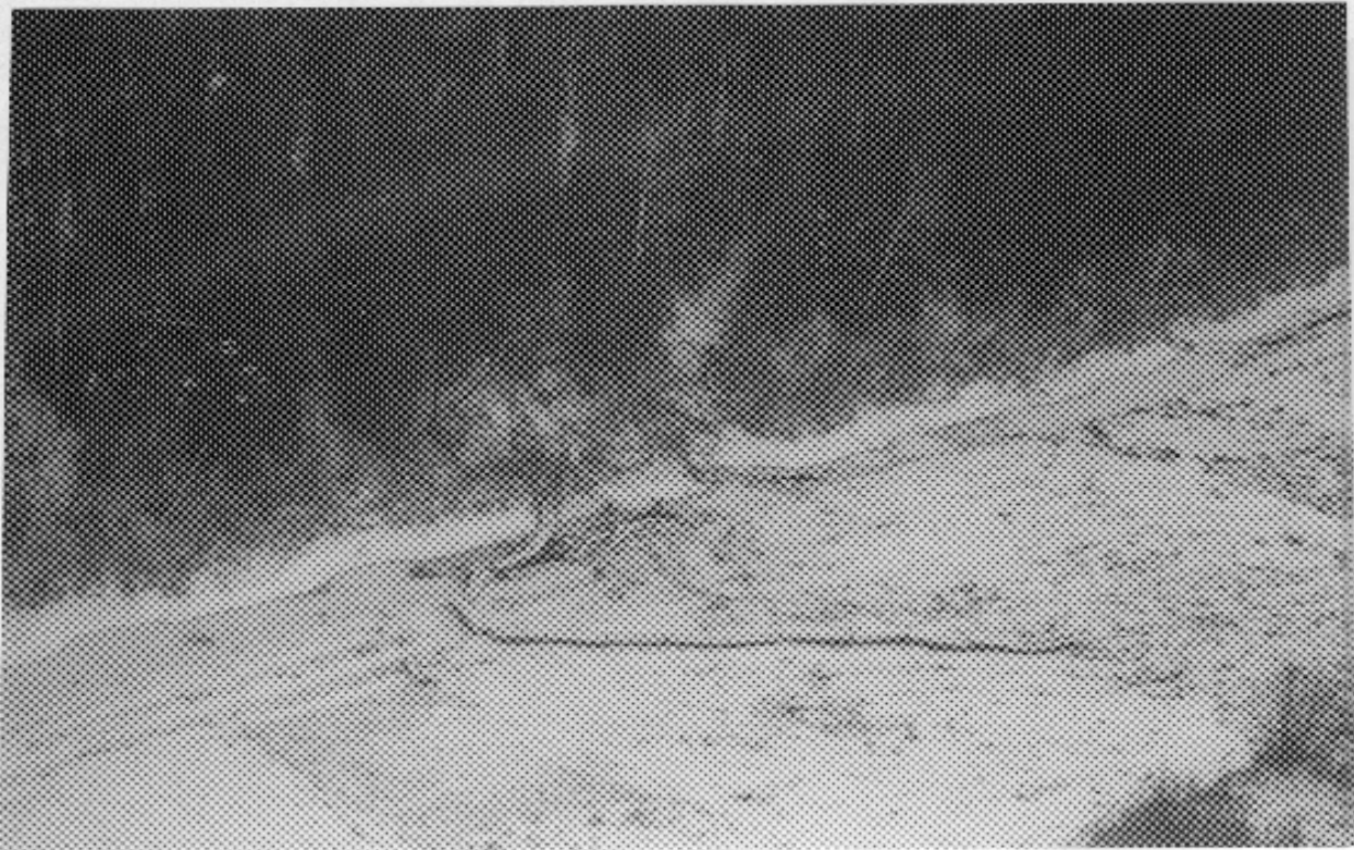
Photo 7: Aerial View of Side Channel Debris Boom (1988) (Note full spanning structure and upstream debris retention in channel.)
