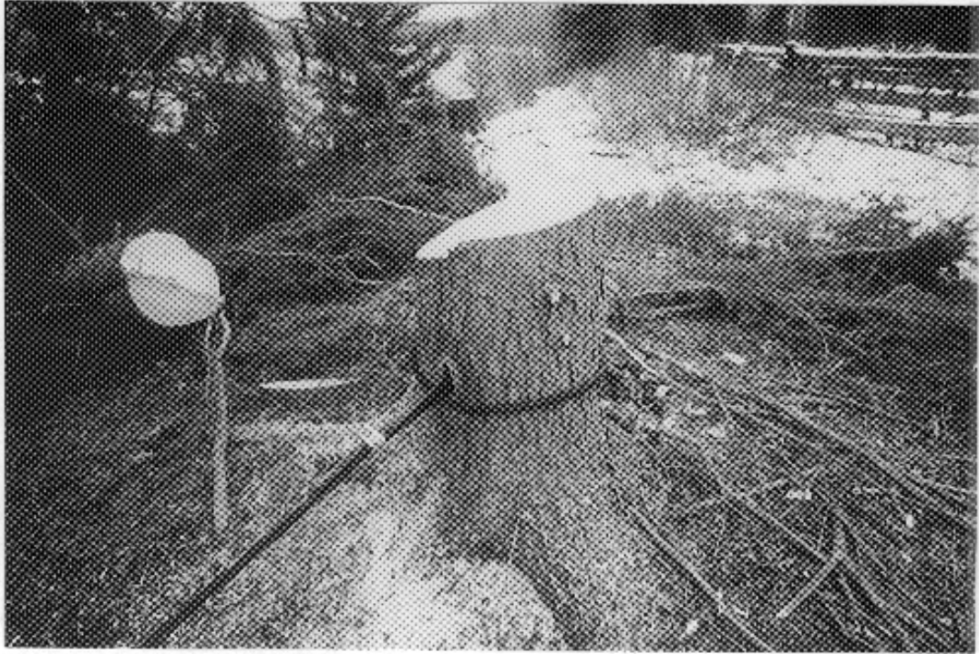
Photo 7: Typical Stump Anchor Cable Attachment Using the Threading and Looping Method (1989 and later)
