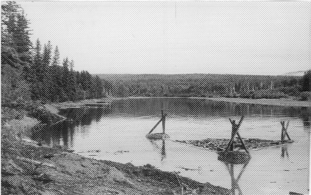
Photo 11: Boomed and Ballasted Channel Jacks (RM25.0CJ), 1989 Seeded With Debris
