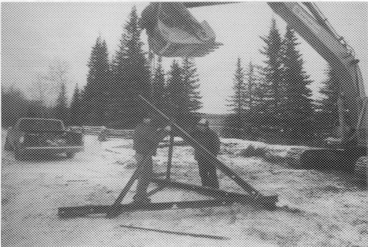
Photo 2: Assembly of Channel Jacks Using Backhoe
