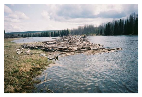
Photograph 15: Rail debris catcher (LM24.2RDC) showing significant debris capture (May 1996).
