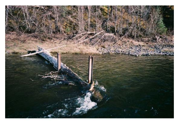
Photograph 13: Rail debris catcher (RM16.5RDC) showing very little debris capture (May 1996).
