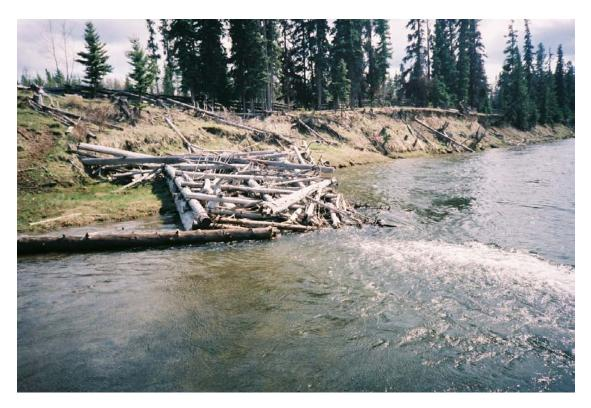
**Photograph 4:** Floating crib (RM27.4FC) not providing much cover as its upstream end pushed onto the shore (May 1996).
