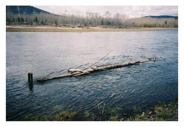
**Photograph 10:** Rail-anchored sweeper (RM26.9RAS) stripped of majority of branches and not providing much cover area (May 1996).
