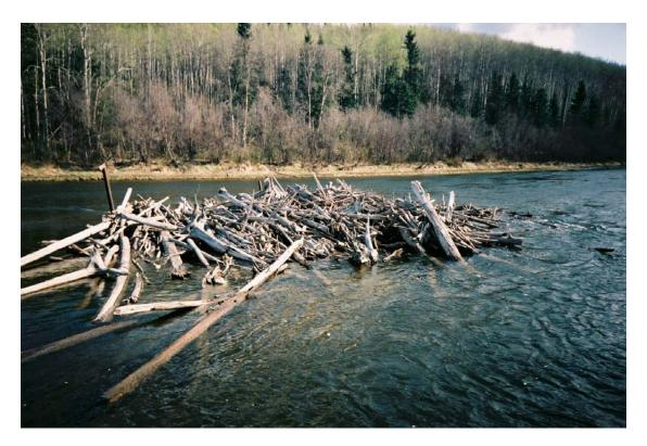
Photograph 12: Large accumulation (180 m<sup>2</sup>) at pipe-pile debris catcher (MC35.4 PDC, May 1996).
