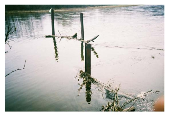
Photograph 17: Break through in the center of the rail debris catcher (RM86.35RDC, May 1996).
