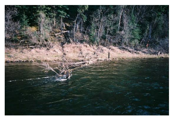
**Photograph 7:** Rail-anchored sweeper (RM16.2RAS) stripped of majority of branches and not providing much cover area (May 1996).
