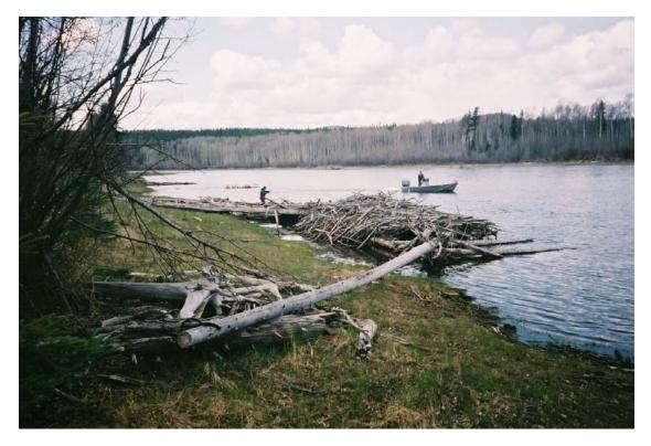
**Photograph 3:** Stable floating crib (RM24.4FC) showing large cover area of 78 m<sup>2</sup> (May 1995).
