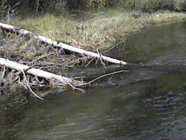
Sept. 8, 1997–LM73..9 Hand Anchored Sweeper (82.6m 3 /s) Constructed in 1991, and modified in 1993 with the addition of a downstream boom, this structure generally fails to trap large woody debris and has deteriorated over time and been reduced in size.
