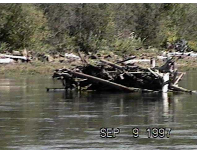
Sept. 9, 1997 - LM24.3 Rail Debris Catcher (82.6m 3 /s) Constructed in 1990, this structure originally did not trap much woody debris, but over time has accumulated material and has remained stable.
