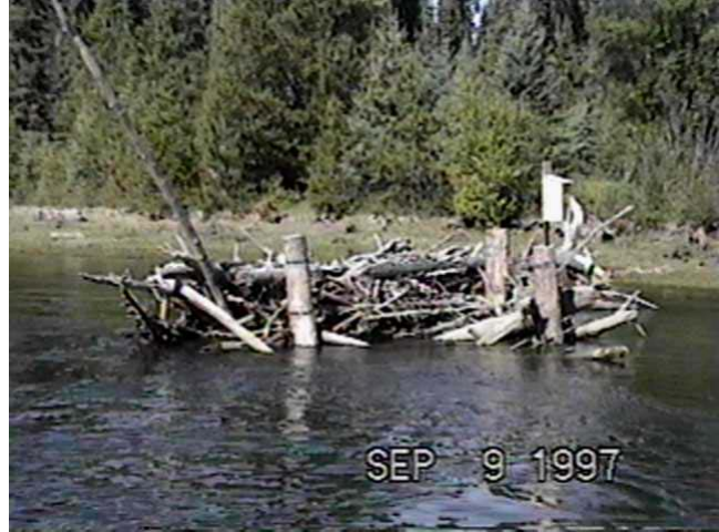
Sept. 9, 1997 - LM21.4 Rail Debris Catcher (82.6m 3 /s) Constructed in 1990, this structure trapped a large amount of debris after construction and was colonized by beavers in 1996.
