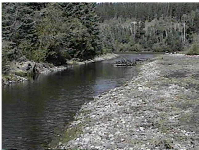
Sept. 9, 1997 - RM17.9 Side Channel (82.6m 3 /s) Constructed in 1988 and modified in 1990 to remove material that was reducing velocities, the side channel currently has extremely low velocities due to a beaver dam at approximately the mid point of the channel.
