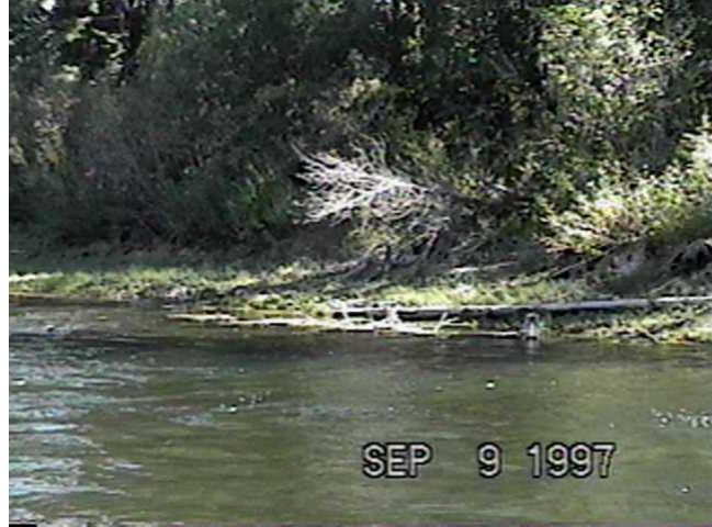
Sept.9,1997-RM22.95 Rail Anchored Sweeper(82.6m 3 /s) Constructed in 1991 this structure is almost completely submerged at high flows and fails to trap woody debris. It has slowly deteriorated in size over time due to defoliation.
