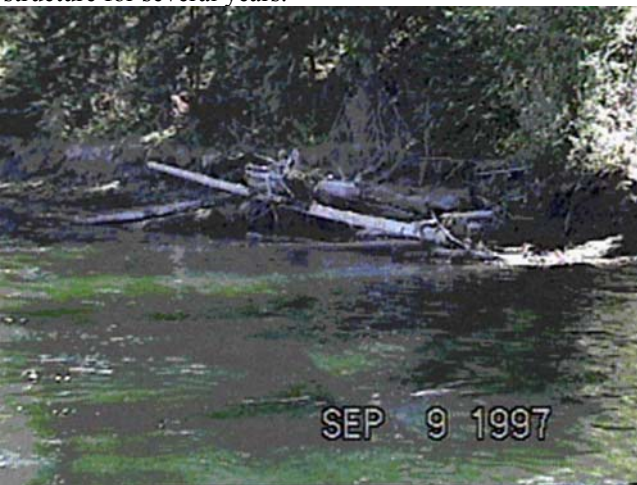
Sept. 9, 1997 - RM28.4 Pseudo Beaver Lodge (82.6m 3 /s) Constructed 1989, this structure fails to trap woody debris despite several efforts at modification and is only creating a very small area of cover. Most debris is on the shore.
