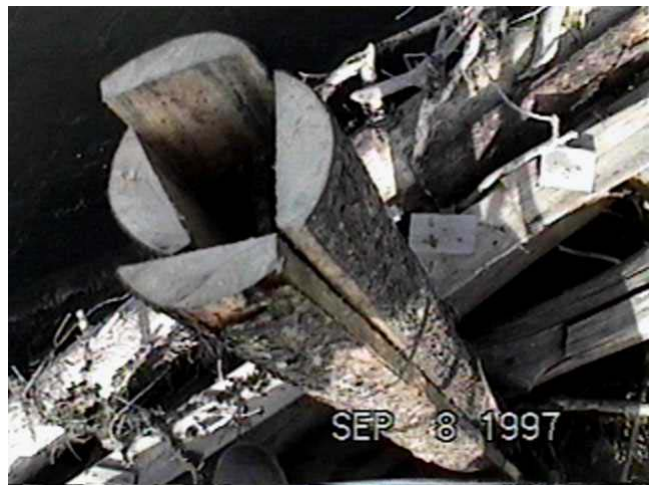
Sept. 8, 1997 – Slab Rail Covers Four slabs were fastened around the rail with banding, or multiple wraps of galvanized fencing wire, and were bolted through the top of the rail to prevent lifting.
