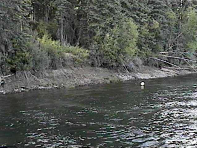
Sept. 8, 1997 – LM82.2 Rail Anchored Sweeper (82.6m 3 /s) Constructed in 1991, this structure generally failed to trap large woody debris, and the entire sweeper was lost in 1997. The rail has been marked to avoid becoming a hazard to navigation.
