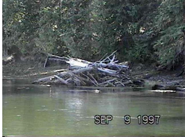
Sept. 9, 1997 - RM24.6 Pseudo Beaver Lodge (82.6m 3 /s) Constructed in 1989, this structure had some success with debris entrapment. It is currently maintaining a small pile of woody debris.
