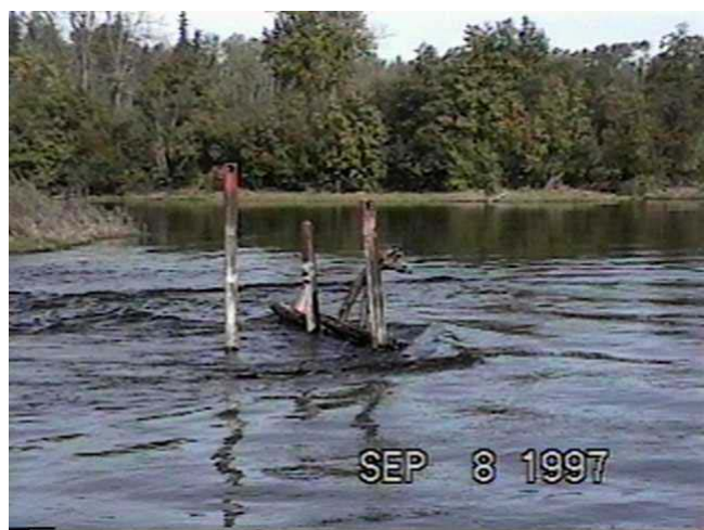
Sept. 8, 1997 – LM 83.0 Rail Debris Catcher (82.6m 3 /s) Constructed in 1991 and modified in 1992, this structure generally fails to trap woody debris, and has slowly been reduced in size over time.
