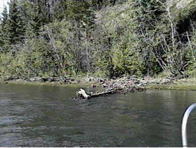
Sept.9,1997-LM 15.6 Rail Anchored Sweeper (82.6m 3 /s) Constructed in 1991, this structure has captured a small amount of debris, and remained relatively stable although some material was lost in 1997.
