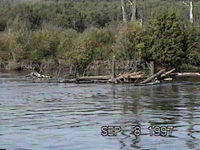
Sept. 8, 1997 – RM86.375 Rail Debris Catcher (82.6m 3 /s) Constructed in 1991, this structure captured a large amount of debris after construction, and subsequently lost some material, but has remained stable and maintains a moderate sized debris pile.
