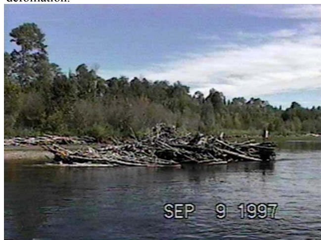
Sept. 9, 1997 - LM24.2 Rail Debris Catcher (82.6m 3 /s) Constructed in 1990, this structure captured a large amount of material after construction and was colonized by beavers several years later. Since that time it has remained stable.
