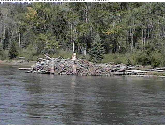
Sept. 9, 1997 - LM18.3 Rail Debris Catcher (82.6m 3 /s) Constructed in 1991, this structure trapped a large amount of debris, and was colonized by beavers immediately after construction, and has remained stable since that time.
