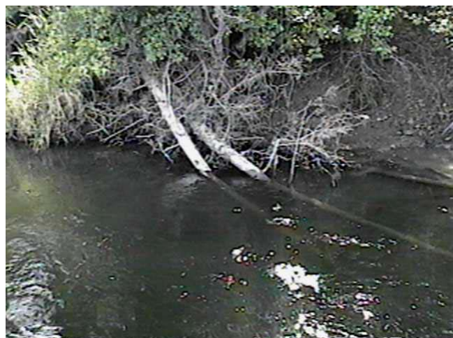
Sept. 8, 1997–LM78.0 Hand Anchored Sweeper (82.6m 3 /s) Constructed in 1991, this structure generally fails to trap large woody debris, and has deteriorated over time, and been reduced in size.
