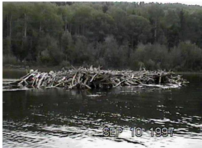
Sept. 10, 1997 -MC35.4 Pipe-Pile Debris Catcher (82.6m 3 /s) Constructed in 1989, this structure captured a large amount of material after construction. It was colonized by beavers several years later and has remained stable.
