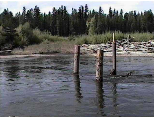
Sept. 8, 1997 – LM80.9 Rail debris Catcher (82.6m 3 /s) Constructed in 1991, and modified in 1997 with the addition of rail covers, this structure has generally failed to trap new debris and was slowly being reduced in size.
