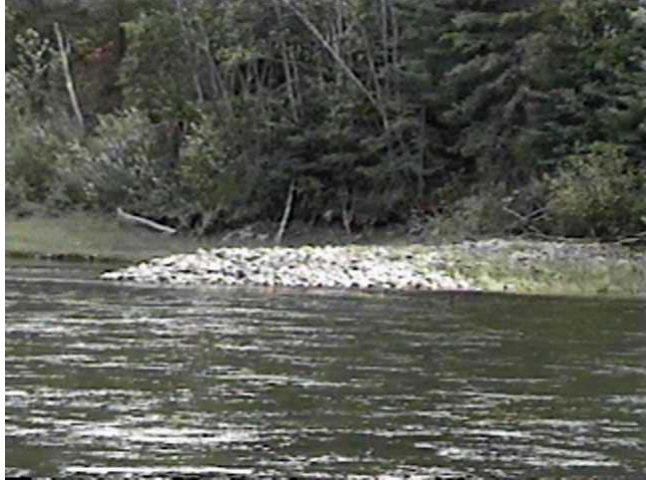
Sept. 9, 1997 - RM17.3 Point Bar (82.6m 3 /s) Constructed in 1989, and modified in 1991, this point bar has remained stable
