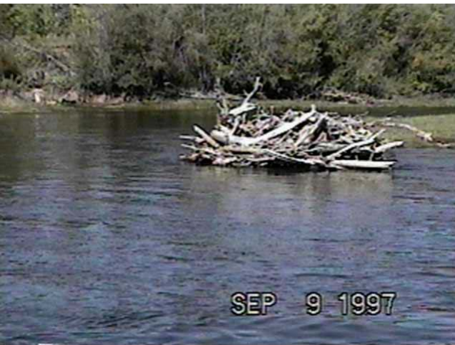
Sept. 9, 1997 - MC25.7 Rail debris Catcher (82.6m 3 /s) Constructed in 1991, this structure has accumulated a small amount of material, and has remained relatively stable over time.
