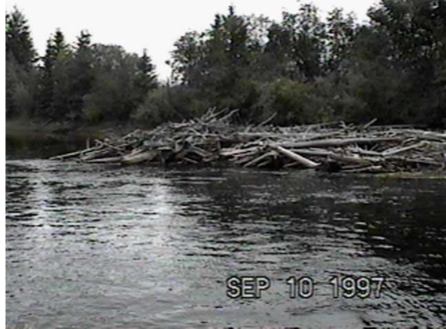
Sept. 10, 1997 - RM28.4 Rail Debris Catcher (82.6m 3 /s) Constructed in 1991, this structure trapped a large amount of debris, and was colonized by beavers after construction, and has remained stable.
