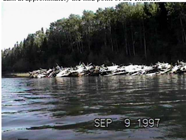
Sept. 9, 1997 - RM20.05 Rail Debris Catcher (82.6m 3 /s) Constructed in 1991, this structure trapped a large amount of debris within the wetted area, and on shore immediately after construction. It has remained stable since that time.
