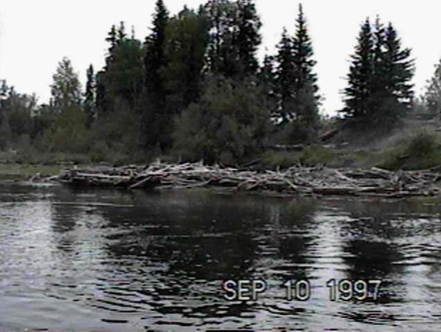
Sept. 10, 1997 - RM27.4 Floating Crib (82.6m 3 /s) Constructed in 1989, and modified in 1991 with additional rail anchors for stability, the failure of the rail anchors, and downstream boom, caused the structure to shift downstream partially on to the shore.
