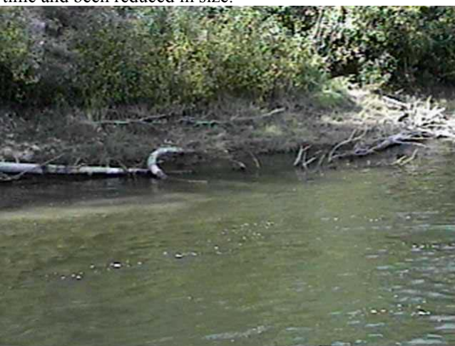
Sept. 8, 1997–LM75..9 Hand Anchored Sweeper (82.6m 3 /s) Constructed in 1991, and modified in 1993 with the addition of a downstream boom, this structure generally fails to trap large woody debris and has deteriorated over time and been reduced in size.
