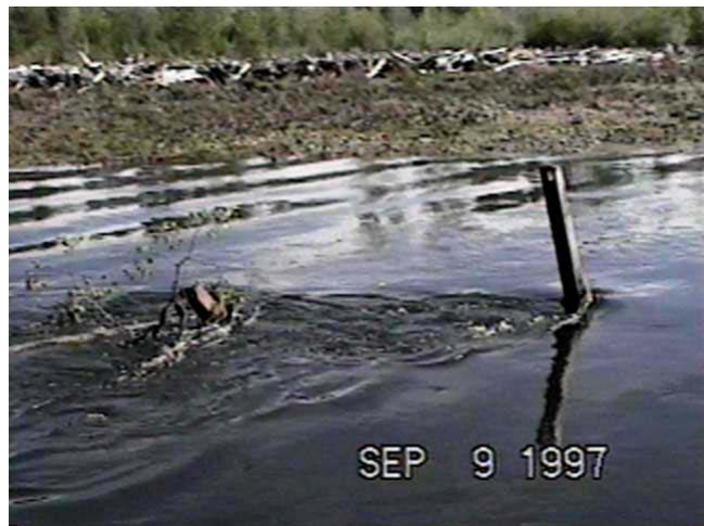
Sept. 9, 1997 - RM25.4 Rail debris Catcher (82.6m 3 /s) Constructed in 1991, this structure captured a large amount of debris after construction. However, scour and high velocities combined to destabilize the rails over time causing the structure to lose most of the woody debris.
