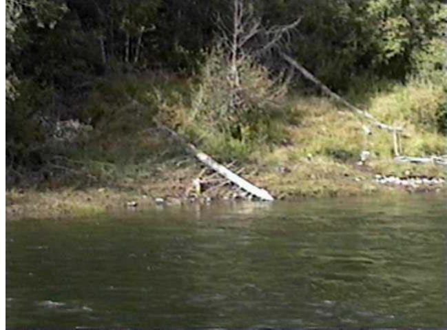
Sept. 8, 1997–LM74.0 Hand Anchored Sweeper (82.6m 3 /s) Constructed in 1991, this structure generally fails to trap large woody debris, and has deteriorated over time, and been reduced in size.
