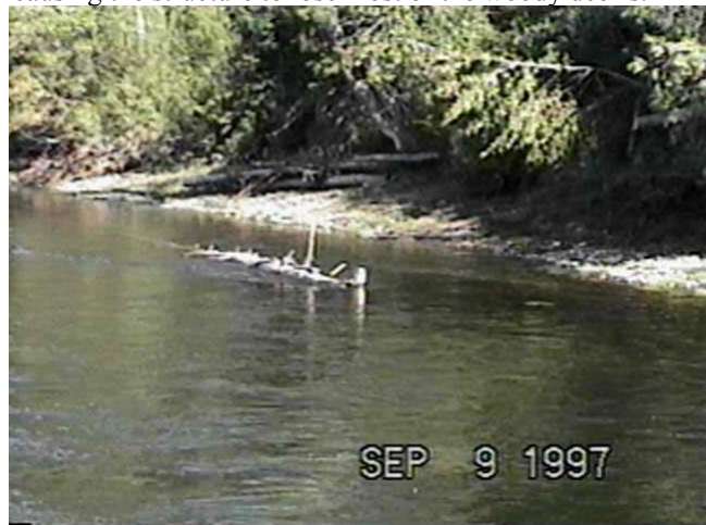
Sept. 9, 1997-RM26.9 Rail Anchored Sweeper (82.6m 3 /s) Constructed in 1991, and modified in 1993, the failure of the modified shore anchor caused the loss of captured material at this complex reducing the structure to a single log attached to a rail.
