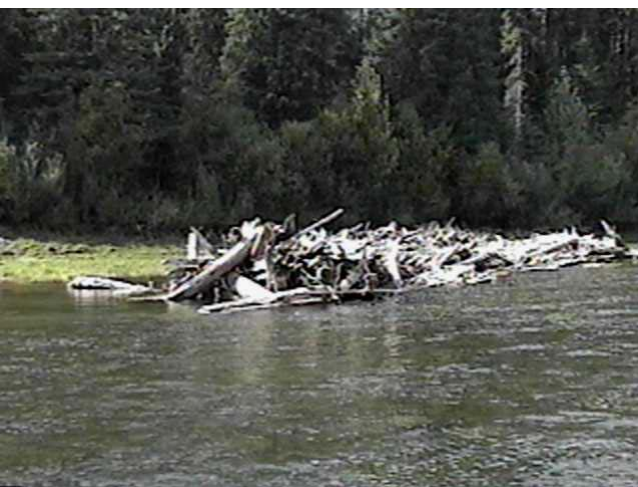
Sept. 9, 1997 - LM17.9 Debris Boom (82.6m 3 /s) Constructed in 1990, this structure prevents excess material from entering the side channel and causing a blockage of flow. It has trapped a large amount of material but is located in shallow water.
