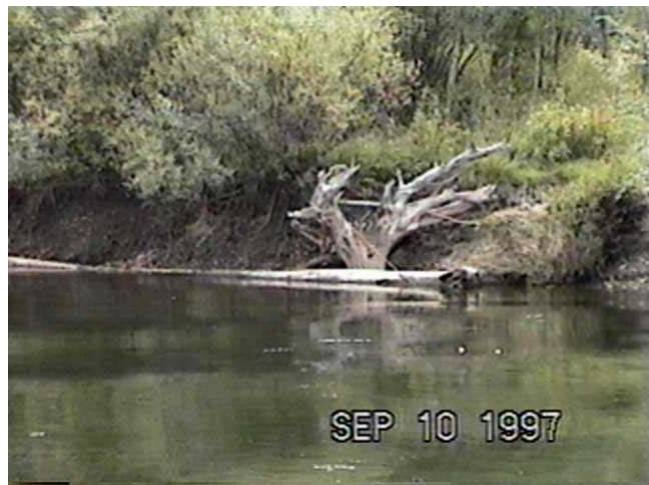
Sept. 10, 1997 - RM31.4 Brushpile (82.6m 3 /s) Constructed in 1988, this structure has not trapped new debris, and the slow loss of and deterioration of seeded material have slowly reduced the size of the structure.
