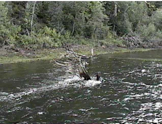
Sept. 9, 1997-RM16.2 Rail Anchored Sweeper (82.6m 3 /s) Constructed in 1991, this structure has failed to capture new debris, and has slowly been reduced in size due to defoliation of the sweeper.
