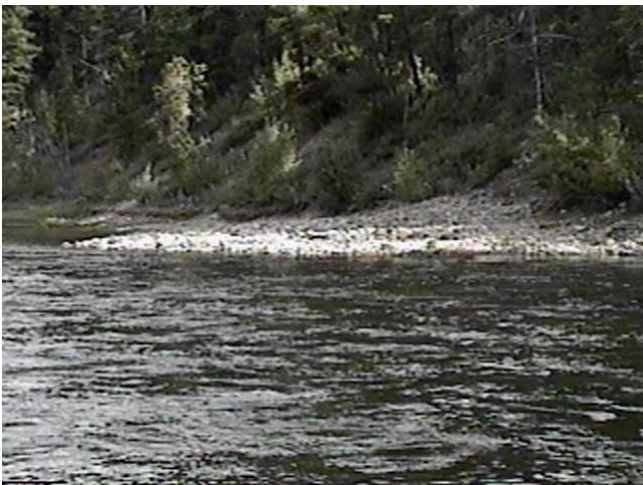
Sept. 9, 1997 - RM17.0 Point Bar (82.6m 3 /s) Constructed in 1989, and modified in 1991, this point bar has remained stable.
