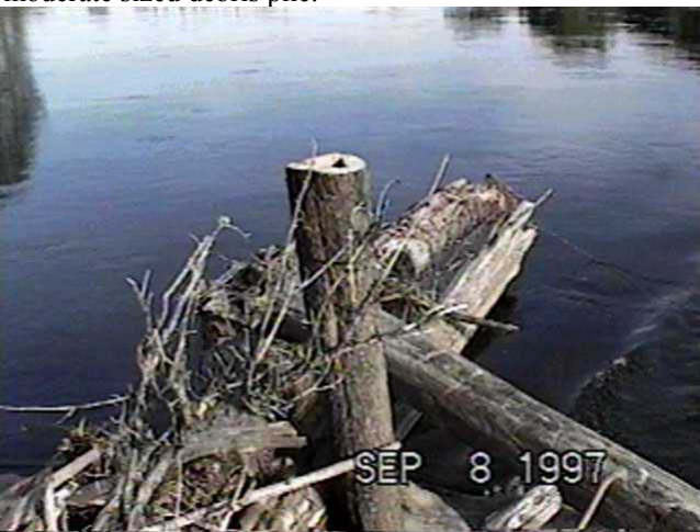
Sept. 8, 1997 – Rail Covers Rail covers were designed and tested in 1997 to improve the esthetics of habitat complexes by giving the rails the appearance of a natural log. V-Groove and slab rail covers were installed on 10 and 6 rails respectively.
