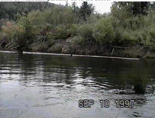
Sept. 10, 1997 - RM3.1 Pseudo Beaver Lodge (82.6m 3 /s) Constructed 1989, this structure fails to trap woody debris despite several efforts at modification, and is creating almost no cover as the structure has been reduced to bare logs.
