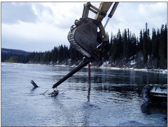
Plate 7. View of the failing downstream rail with the wooden top casing being removed.
