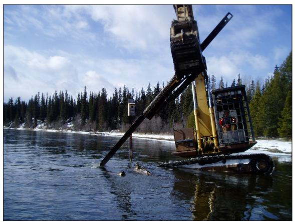
Plate 8. View of the failing rail that was furthest from shore being removed.
