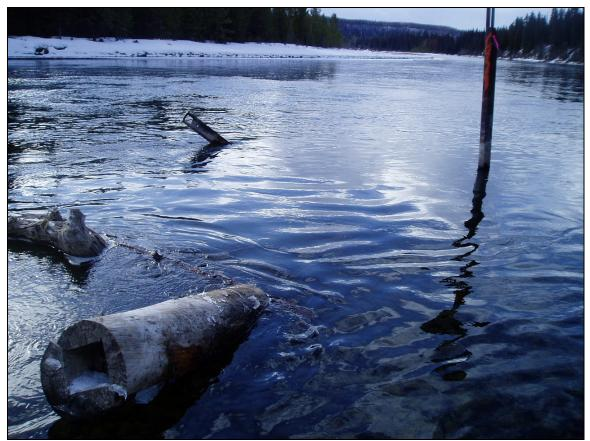
**Plate 1.** Upstream view of the condition of the rail debris catcher on February 22, 2005 prior to being removed. Note the angle of the outer rail and the downstream rail (with wood casing).
