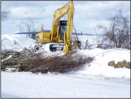
**Plate # 3. Date:** December 21, 2006. **Comments:** Showing the small woody debris installed along the bank edge, and the operator clearing the tracks prior to crossing.
