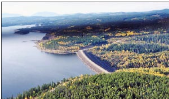
Kenney Dam and Nechako Reservoir
